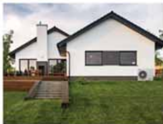
Air Source Heating
