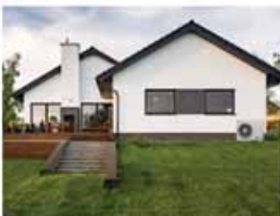
Air Source Heating
