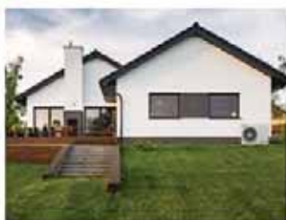
Air Source Heating
