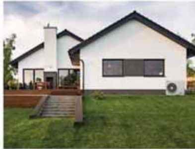
Air Source Heating
