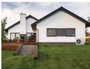
Air Source Heating
